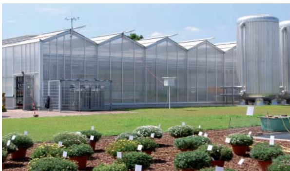
ZINEG Versuchsanlage in Hannover-Ahlem
